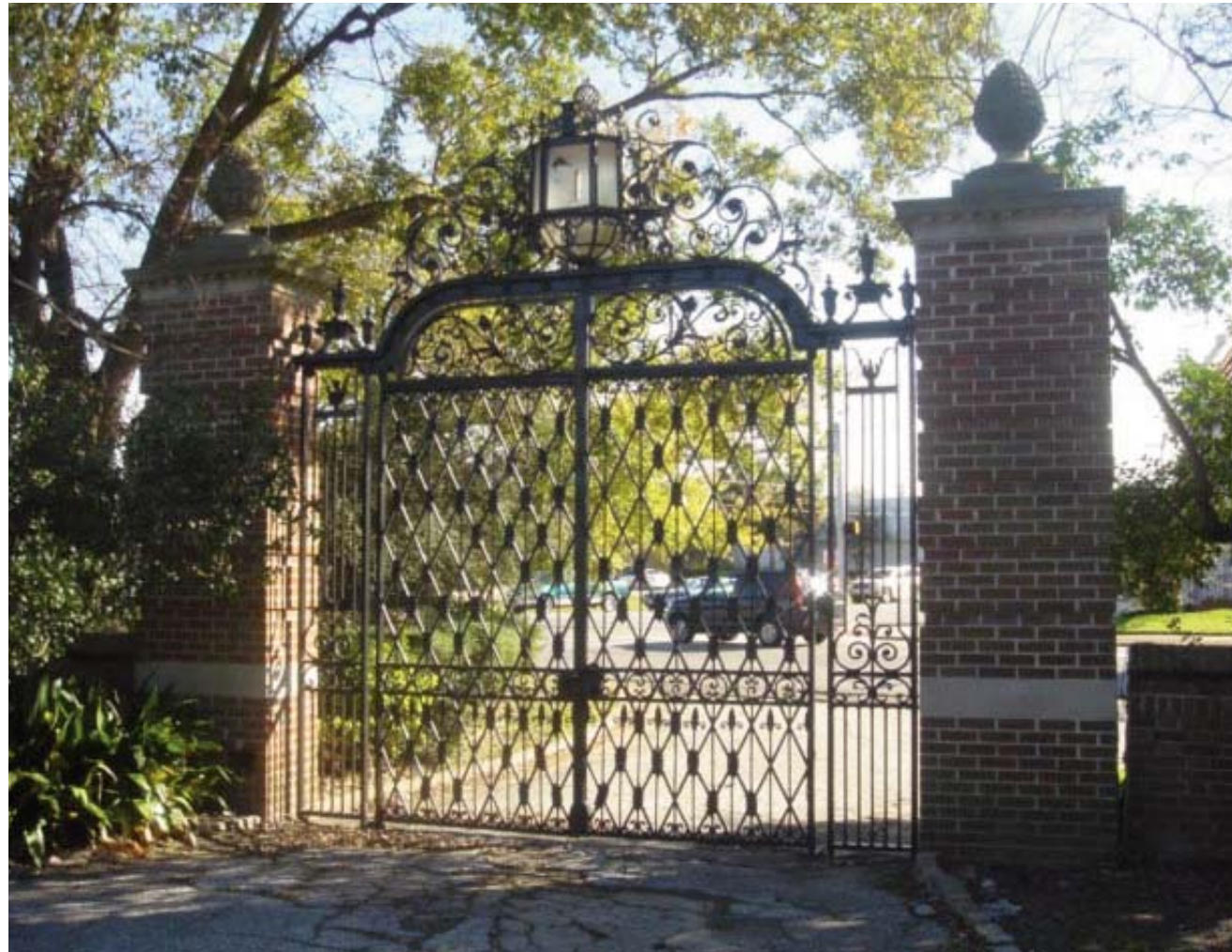
Original south gate facing Calder Avenue
